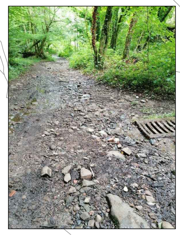
Existing gully to be jetted and raised to new levels
